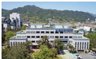
01 1호관(본관) Main Building(1)
